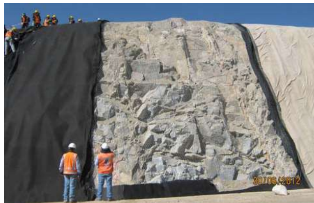
Figure 3: Very steep rocky slope with irregular shape after blasting
