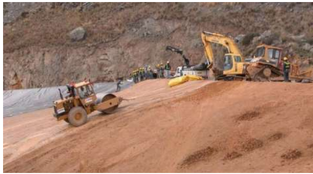
Figure 5: Soil liner compaction on a very steep slope
