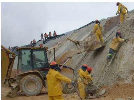
Figure 4: Typical grading and protection for geosynthetics installation on very steep slopes
