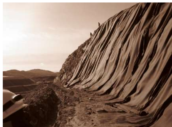
Figure 4: Typical grading and protection for geosynthetics installation on very steep slopes
