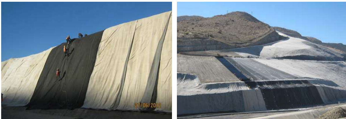
Figure 8: Complex geomembrane and GCL liner installation on very aggressive terrain
