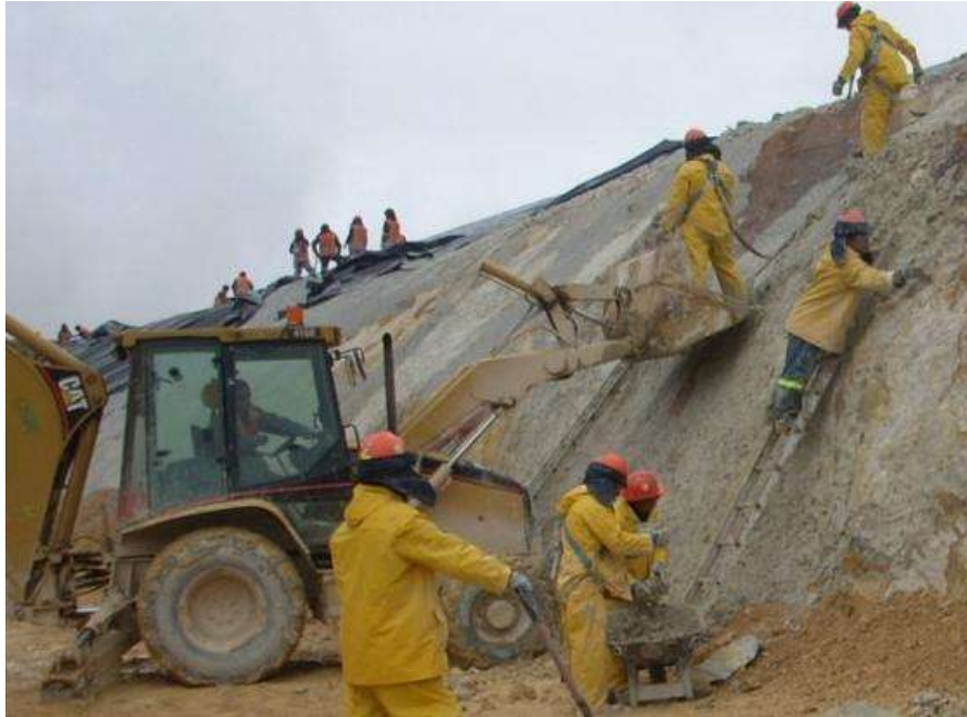
Figure 1: Surface preparation before GCL and geomembrane installation
