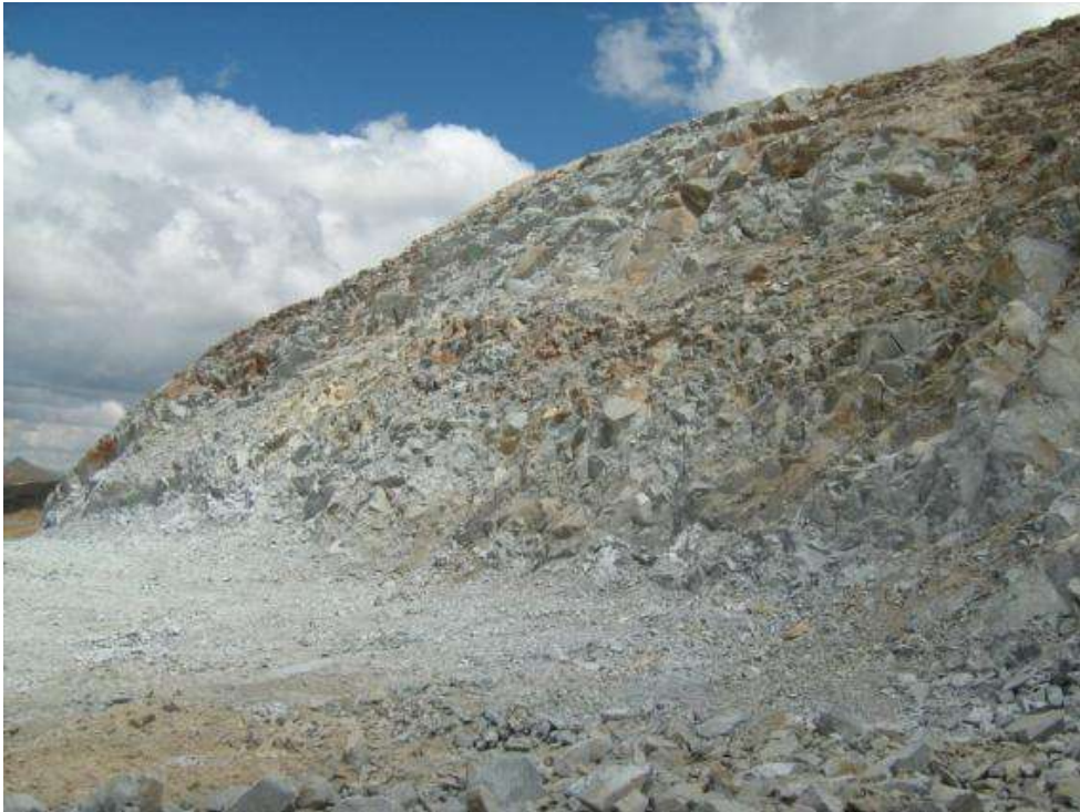
Figure 5: Protection must be included in sharp slopes in order to avoid damage to the GCL
