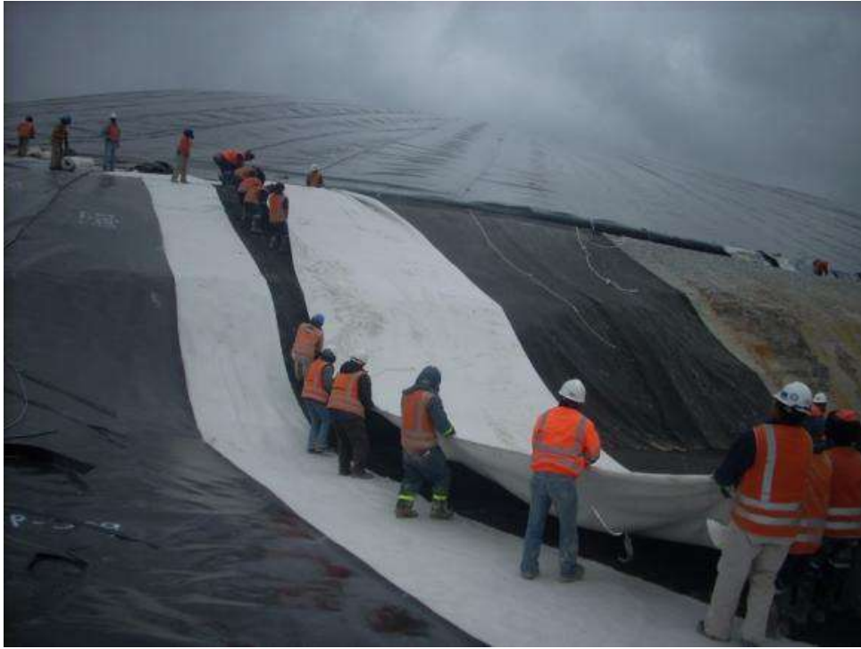
Figure 4: Geocomposite, GCL, and geomembrane installation
