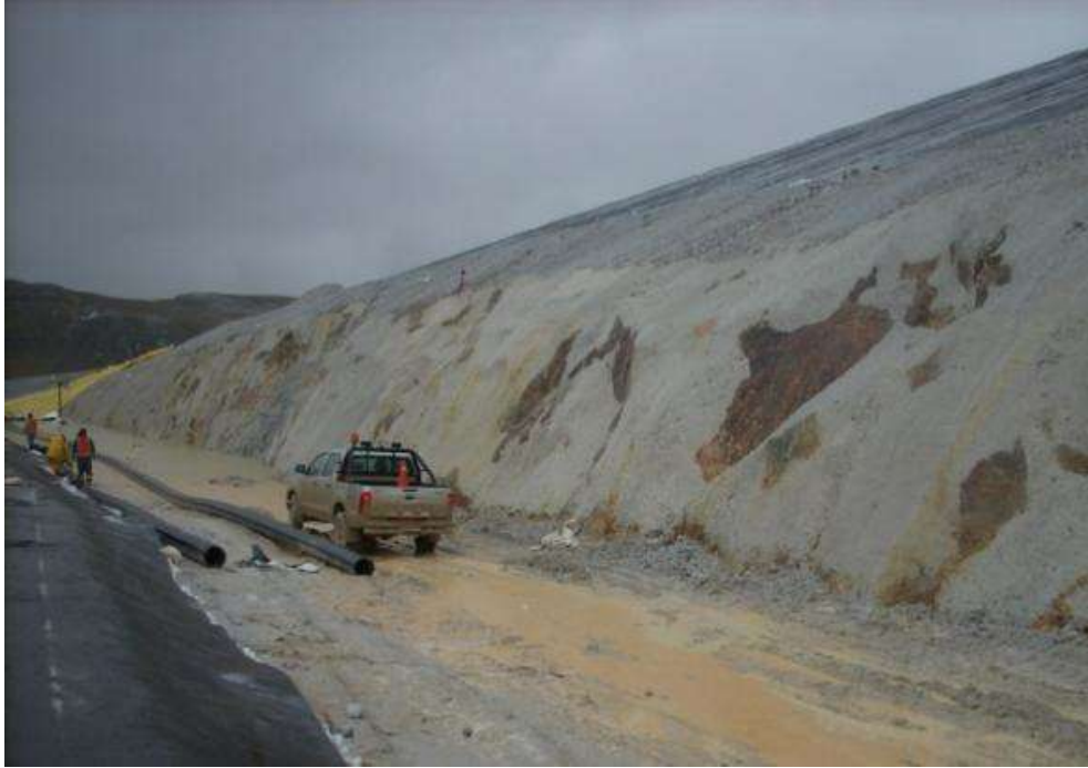
Figure 3: Surface prepared before GCL and geomembrane installation
