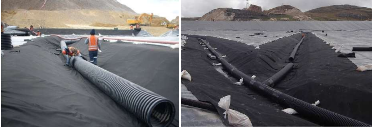
Figure 10: Main header installation works in trenches
