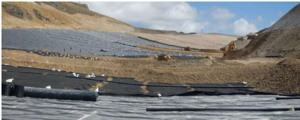
Figure 5: Non-woven geotextile placed for geomembrane protection
