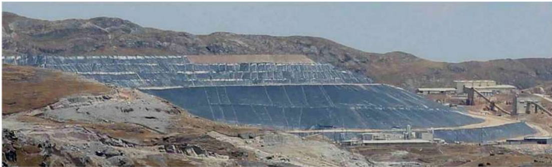
Figure 1: Very deep heap leach pad in the Peruvian Andes
