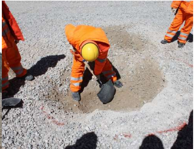
Figure 8: Overliner excavation
