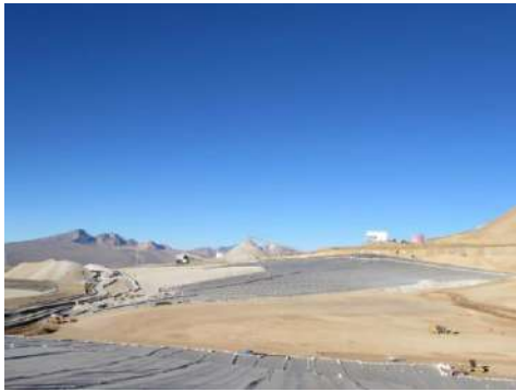
Figure 4 Site # 1 General View of exposed geomembrane liner to be surveyed, perimeter berms and previous phases
