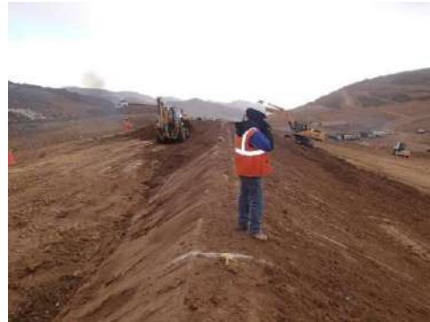
Figure 5 Site #1 Perimeter Berm and Soil Line, prior to liner installation
