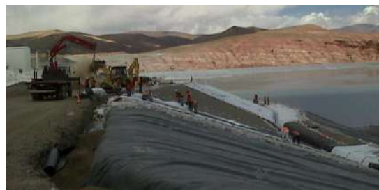
Figure 7 Site #2 Geomembrane liner and GCL installation
